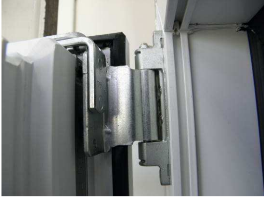
Fig. 5 Tilt mechanism pivot, rebate view
