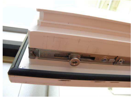
Fig. 12 Locking situation, casement member 3
