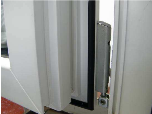
Fig. 7 Corner pivot, rebate view
