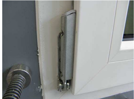
Fig. 8 Corner pivot, internal view
