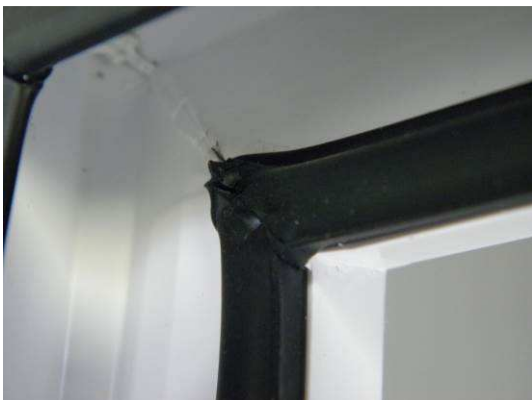
Fig. 2 External rebate seal, corner design
