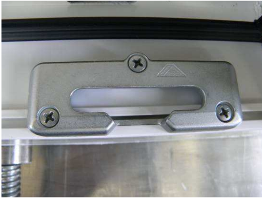
Fig. 11 Locking situation, frame member 3
