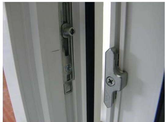
Fig. 10 Locking situation, frame member / casement member 2
